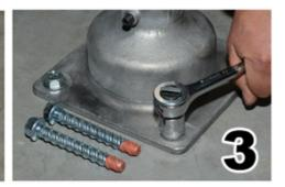
Place the base plate over the four holes and use a socket wrench or high speed drill with a 3/4" drive to thread all four bolts
